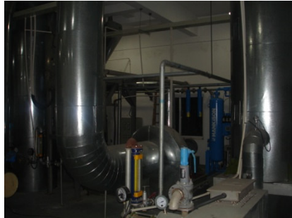
On the very top floor of the building, the raw material is mixed and extruded
